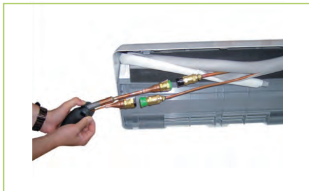
Fig. 37: Installation on the indoor unit
