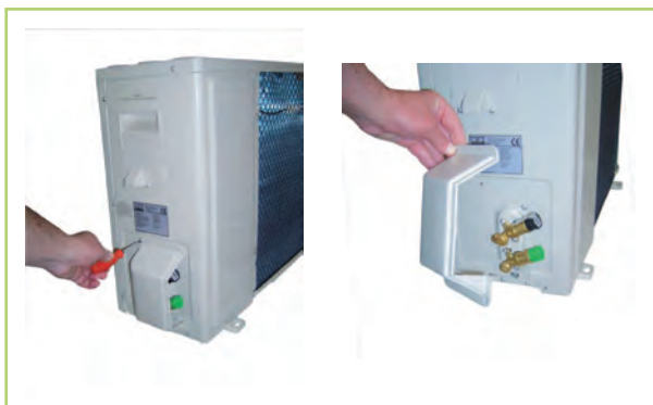
Fig. 32: Remove the plastic cover
