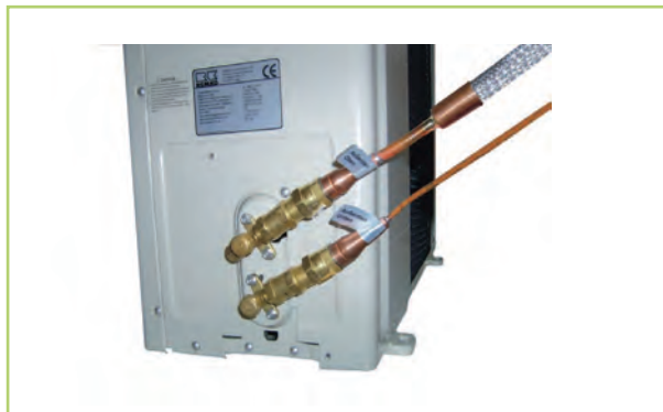
Fig. 36: Installation on the outdoor unit
