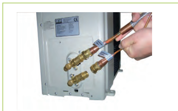
Fig. 35: Position of the quick-release couplings
