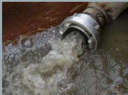
■ Step 3: Start pumping
